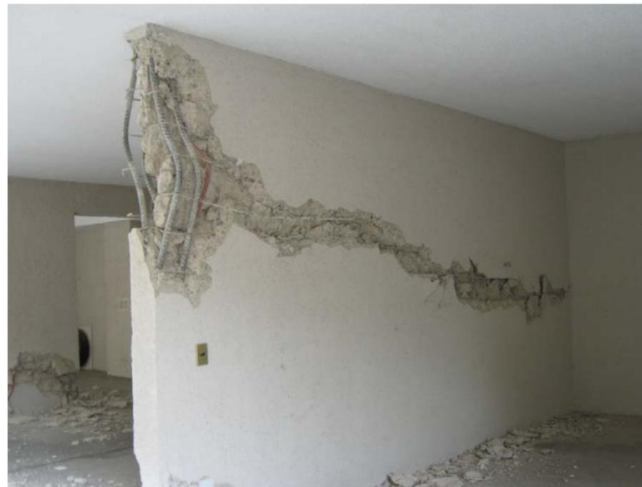
Figure 5-5 Cracking, spalling, crushing, and bar buckling in the transverse shear wall on Line 9 (photo courtesy of Patricio Bonelli).
