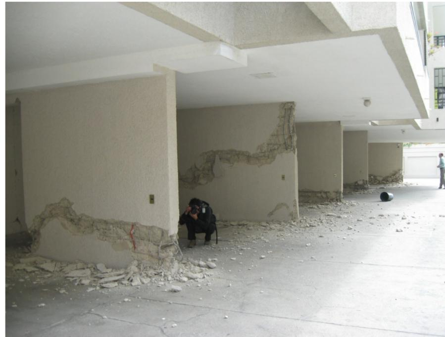
Figure 5-4 Overall damage sustained in the first-story transverse shear walls of the case study building (photo courtesy of Patricio Bonelli).
